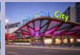
Northpoint City North Wing
